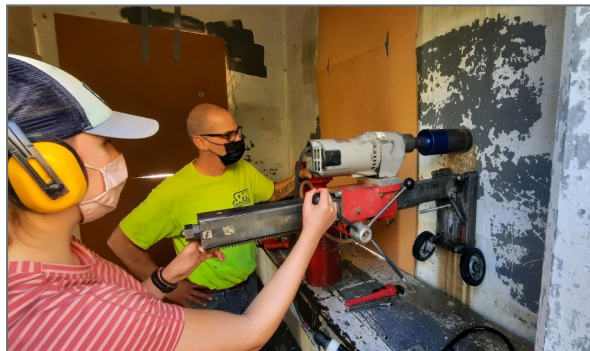
SHN materials specialists sample concrete at the Punta Gorda lighthouse.
