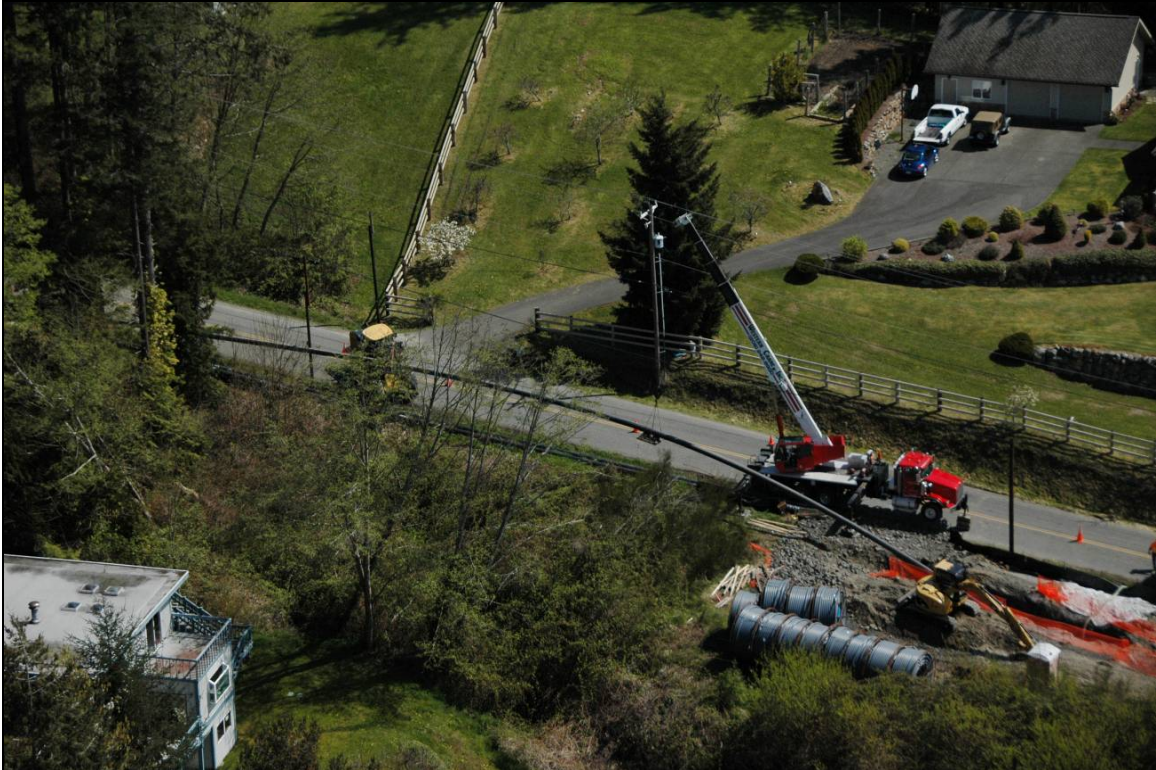
Figure 7 – Roping in Steel Casing During Pullback
