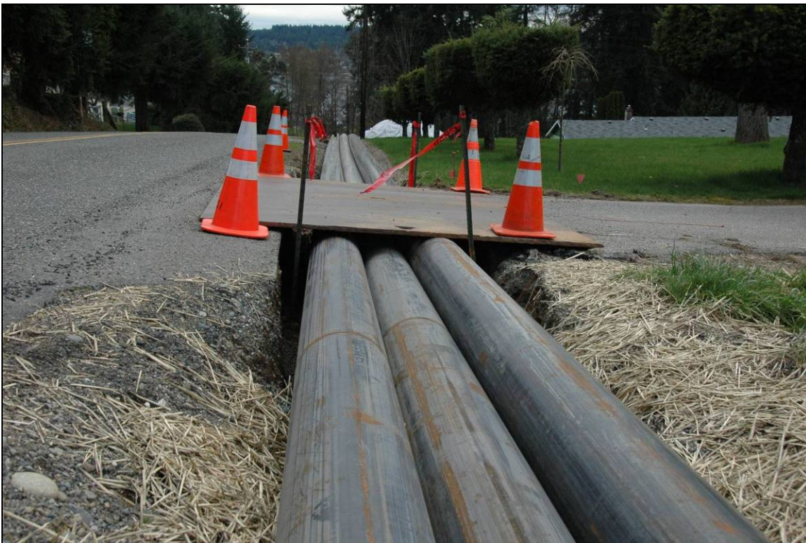
Figure 5 – Lay down of 12-inch Steel Casing
