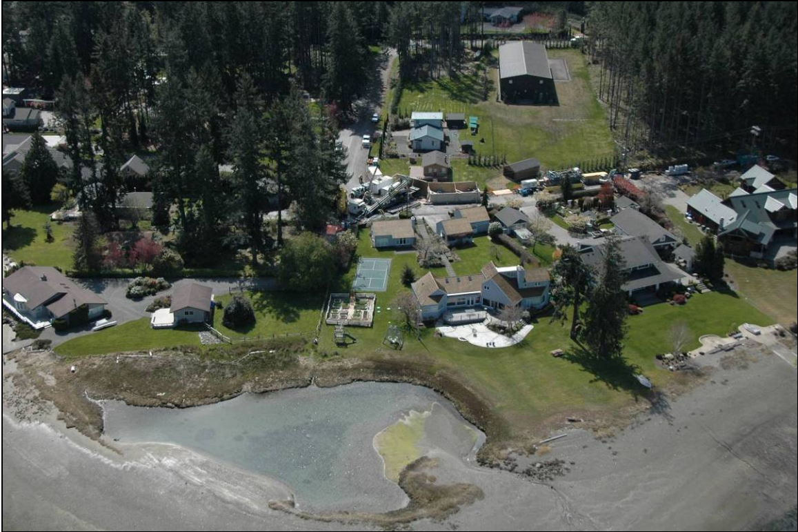
Figure 4 – HDD Entrance on Fox Island side
