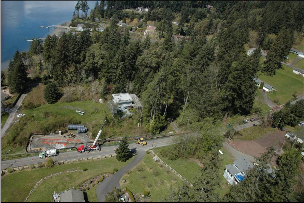
Figure 3 – HDD Exit on peninsula side
