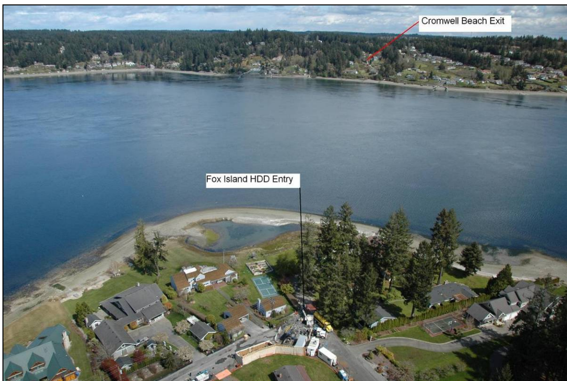
Figure 8 -Fox Island Cable Crossing Project Entry and Exit Locations
