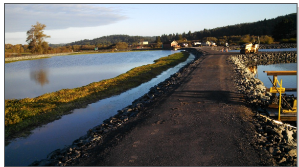
Wastewater treatment ponds for the City of Blue Lake, CA
