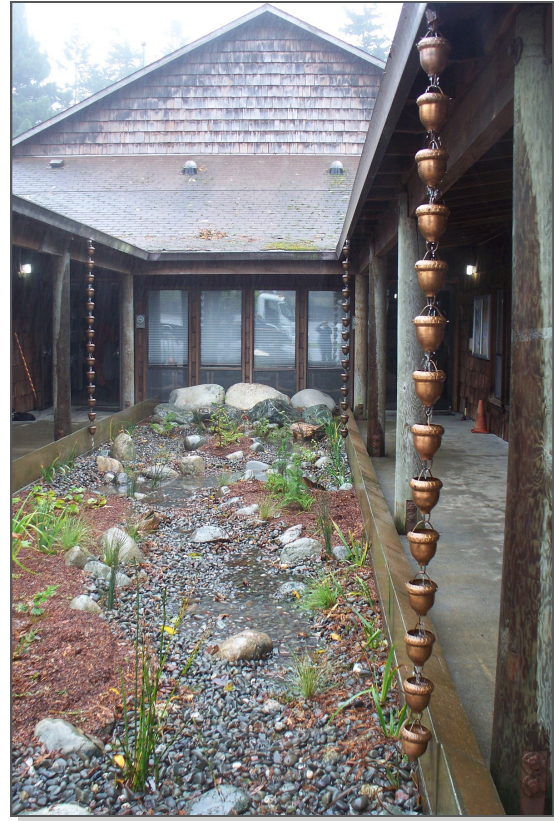
A low impact development rain garden, Trinidad Rancheria, CA
