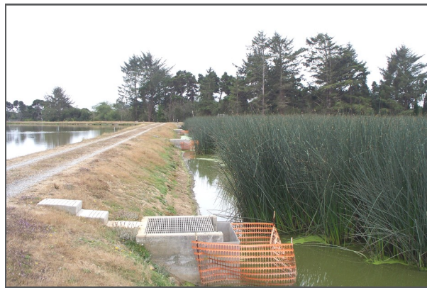
Wastewater treatment via a natural pond system in McKinleyville, CA
