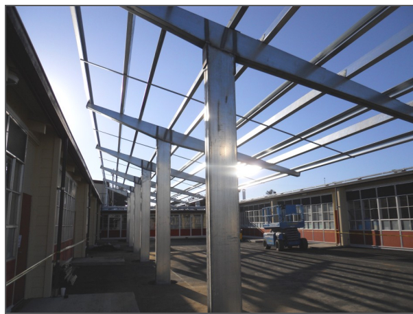
Racks for a solar panel array at Fort Bragg High School, Fort Bragg, CA.
