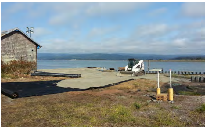
EPA strike team installing cap and placing clean fill at the site.
