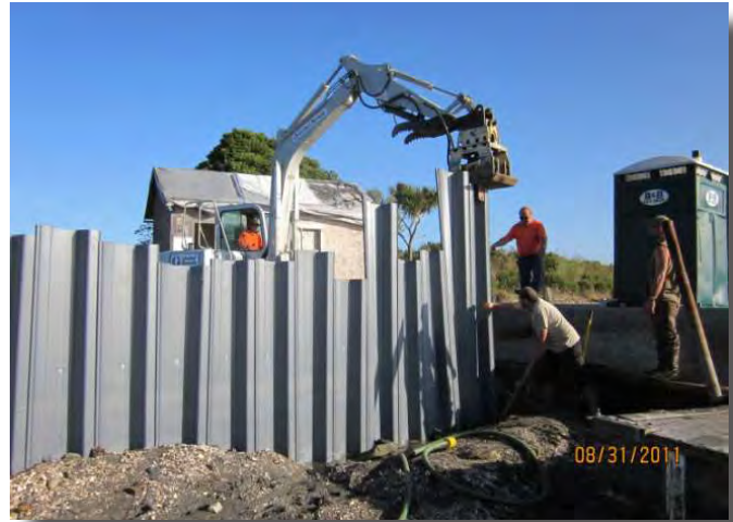
A total of 220 linear feet of sheet pile at the site prevents erosion, protecting the shell midden and other cultural and environmental resources.
