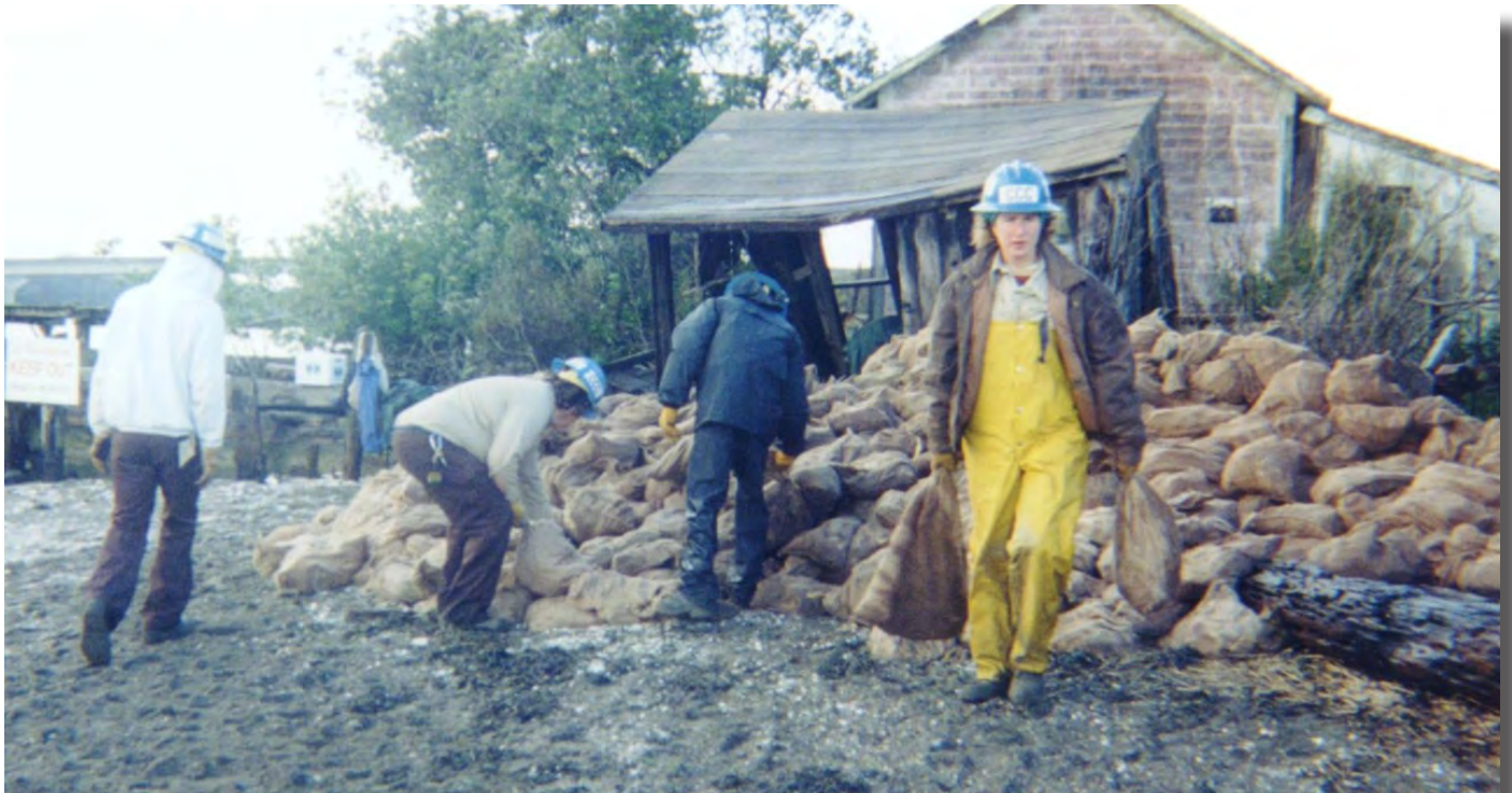
Workers using oyster shells for erosion control.
