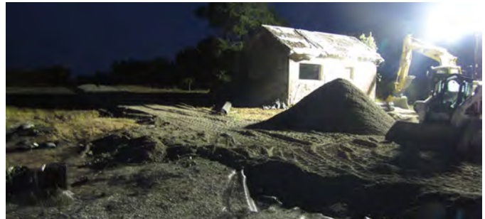
Due to tidal limitations, EPA worked around the clock to cap the site.
