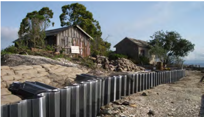
Sheet pile installation and bulkhead repair activities in 2011.
