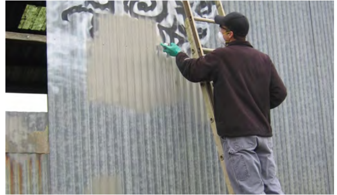
Tim Nelson removes graffiti from the Butler Building.
